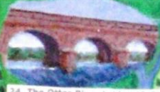
24. The Otter River bridge (& Ford) 1 st 1259, pres. 1840
